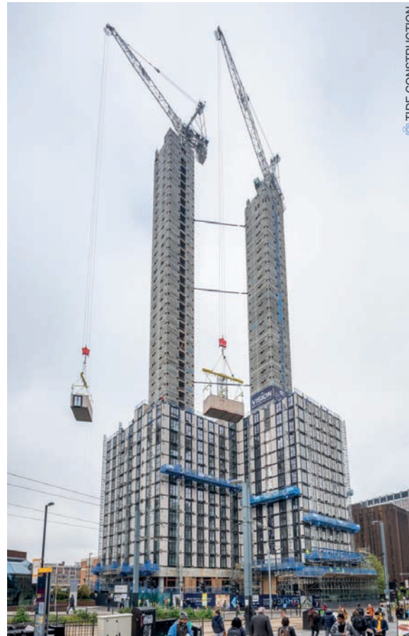
FIGURE 2: Volumetric modules being lifted into place around reinforced concrete cores during construction of Ten Degrees
