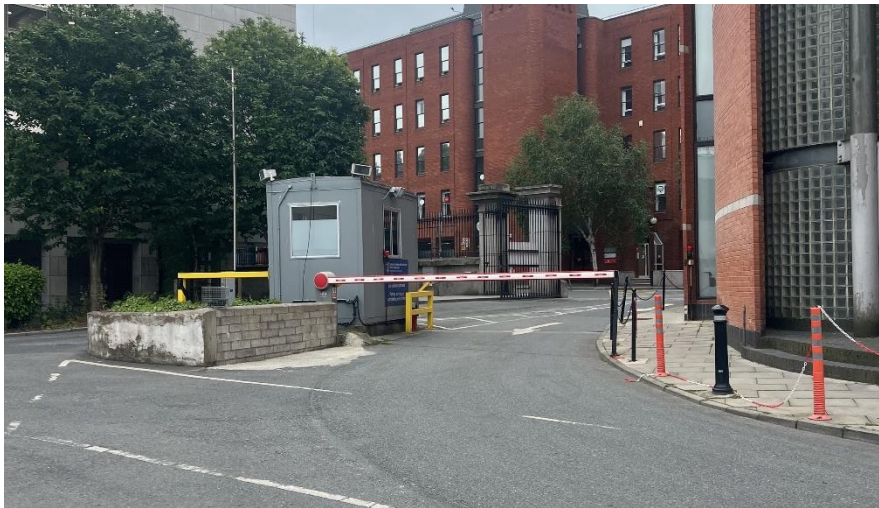
Figure 6-5 Vehicle Barrier at Lincoln Place Gate
