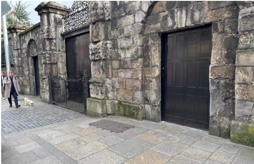
Figure 3-9 Wide Footpaths at Grafton Street
